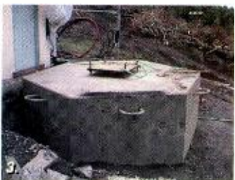
Le Blanc Broadcast is building a new tower for KGW(TV) Portland, Ore., that will also house KOBP's NTSC and DTV antennas: 1. Inside tower's guy anchor. 2. KGW's new Dielectric antennas. 3. A concrete base. 4. A steel base that will be mounted atop the concrete base.
